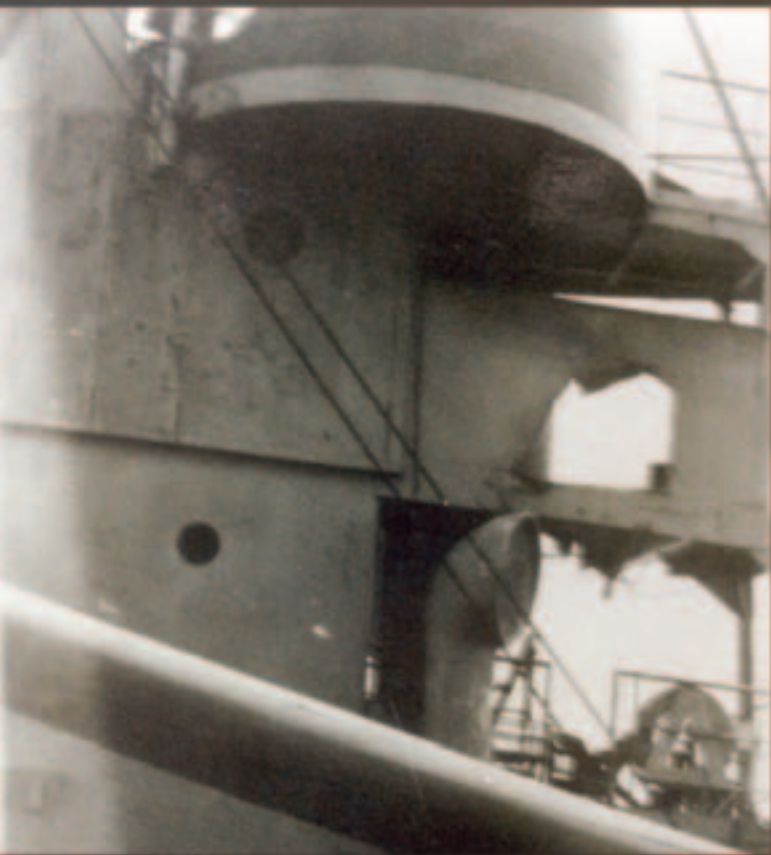
Damage visible on the Marcus Daly after the attack on Dec 10, 1944.
